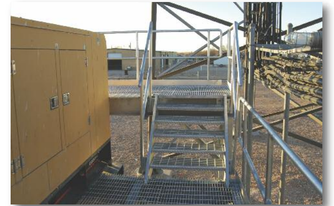
Custom stairs and railings help meet OSHA requirements.
